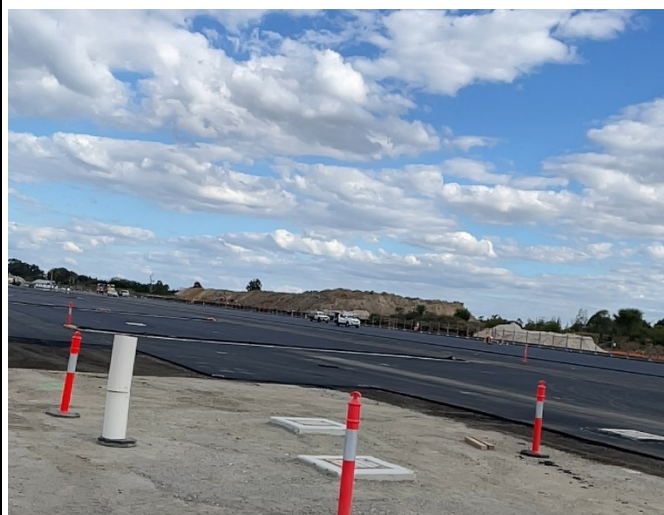
Paved container storage area showing large stockpiles in background.
