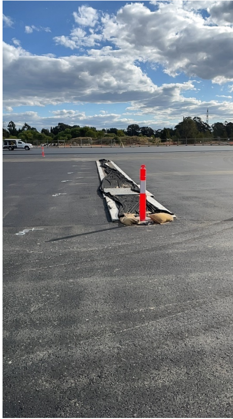
Completed covered drainage pits
