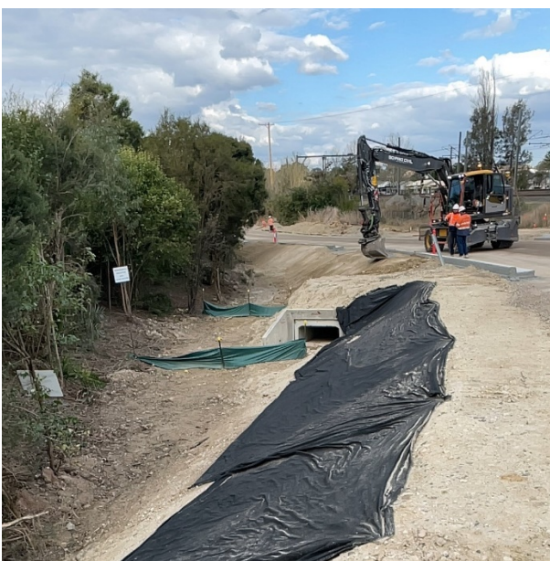
Approved entrance road showing erosion controls and kerbing installation
