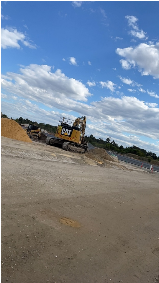
Stockpiling of temporary material
