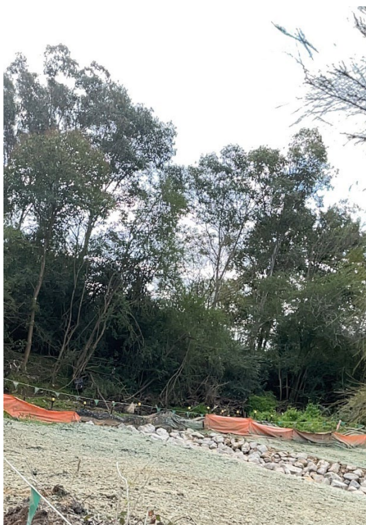
Basin outlet showing scour protection and end of line control
