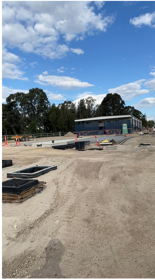
Near completed office/administration
