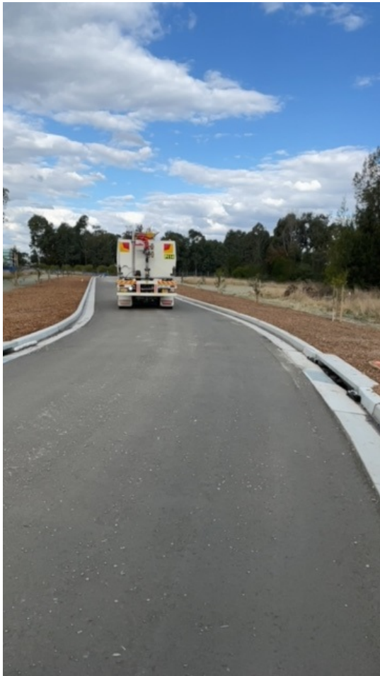
Site entry from Lee Holmes Drive
