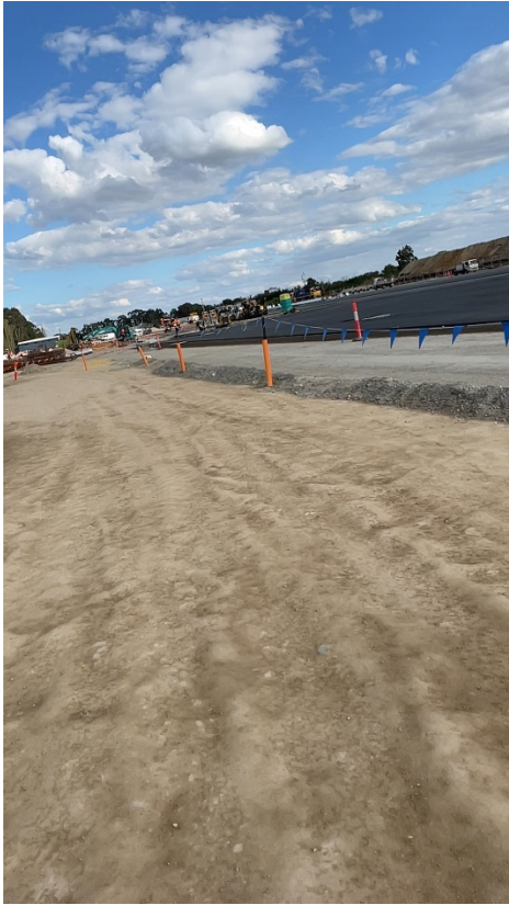
Container storage area sealing in progress
