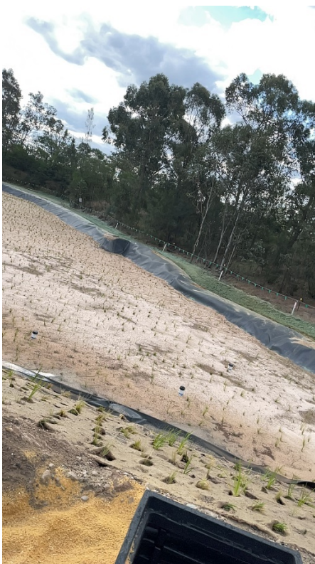
Basin showing planting and hydromulching
