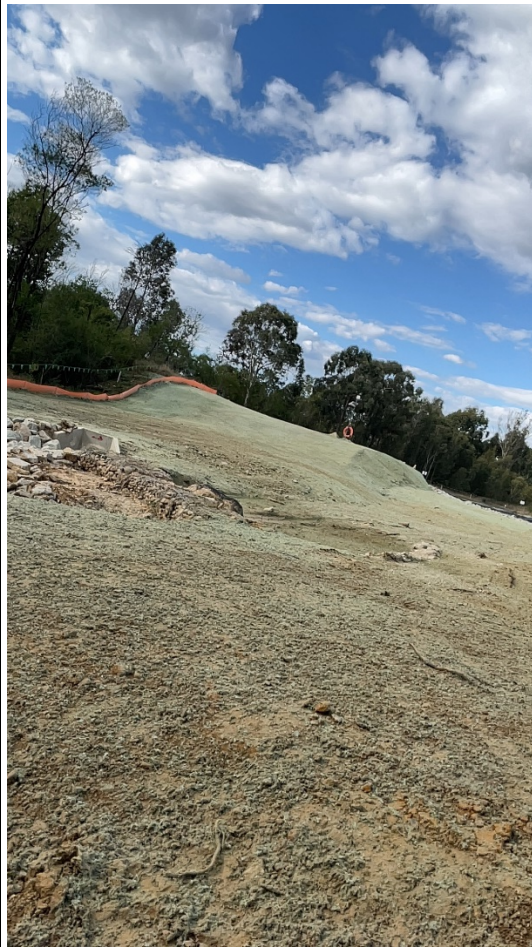
Delineation of site and erosion control
