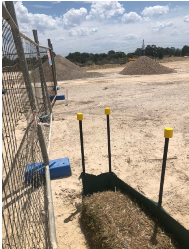
Delineation of site and erosion control
