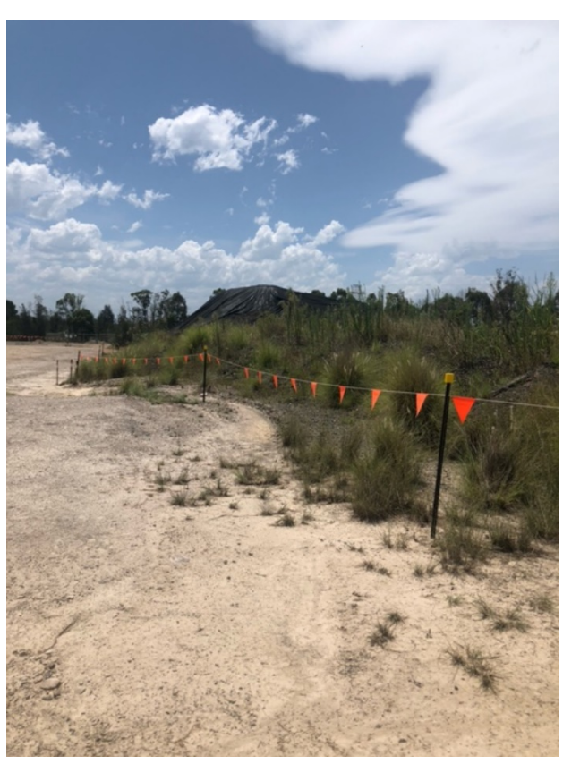
Delineation of site and covered stockpile
