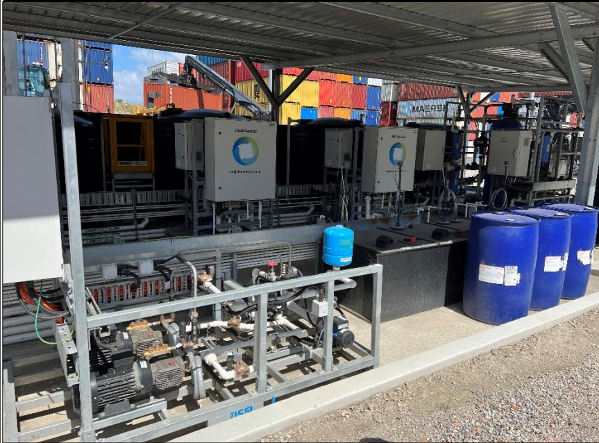
PHOTO 3: CLEARWATER WASTEWATER TREATMENT SYSTEM
